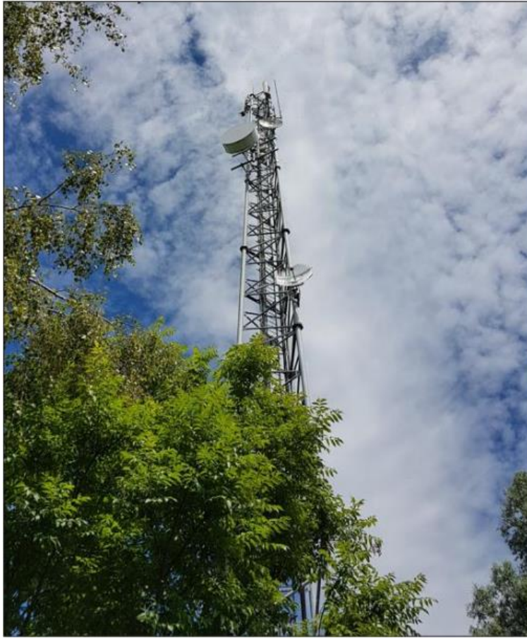
Fig. 1 - 36 metre lattice structure located at Derrygreenagh ('Cellnex Ireland mast'.
